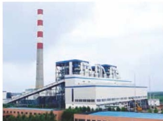
Chipping Xinyuan Aluminum 700 MW unit, the first 500 kV integrated and first thermal power project of the Group
