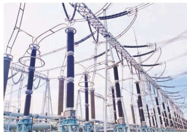
Shanxi Beiyue 1000kV Substation Project
