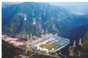
Changji-Guquan ±1,100 kV DC Transmission Project
