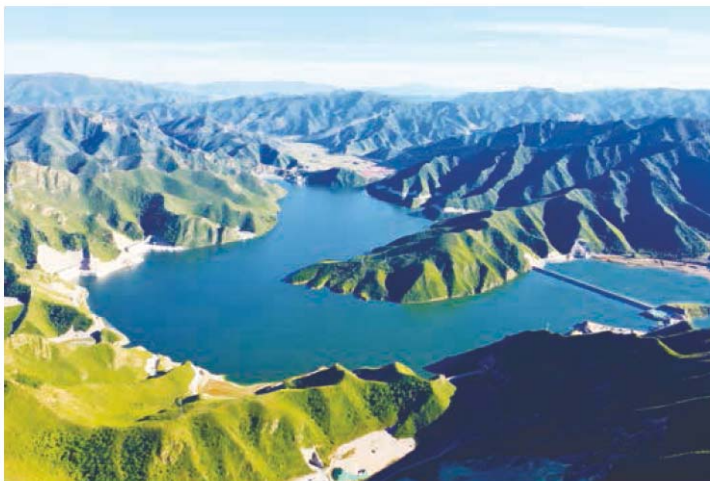
Hebei Fengning 3,600 MW pumped storage power station, the world's largest pumped storage power station, a key project for Beijing 2022 Winter Olympics
