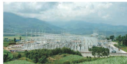
400kV Soyo-Kapary Complete Project Phase I in
