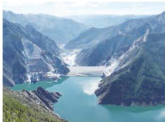
3,000 MW Sichuan Yalong River Lianghekou Hydropower Station, the project with the highest shaft height of the Group (254 m)
