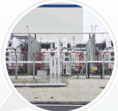
DFP-450000/500 transformer, used in Karachi nuclear power project in Pakistan
